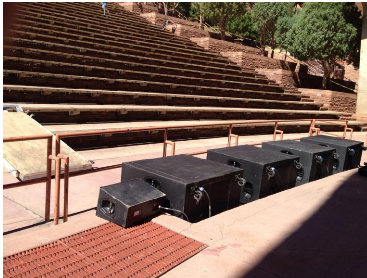
Vibration measurement location in the amphitheate
